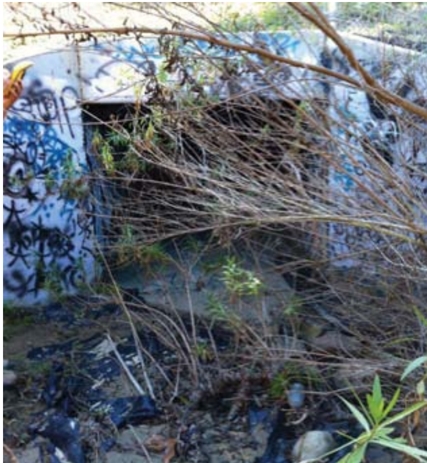
Photo 10 – Photo depicts the culvert into which Ruffin and Sandrock Canyons drain. This culvert flows under the Escala Community and empties into the San Diego River. Photo facing south.
