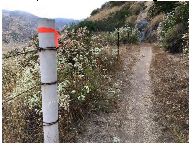
Figure 1. Image of asbestos pole and barbed wire along Flume Trail
