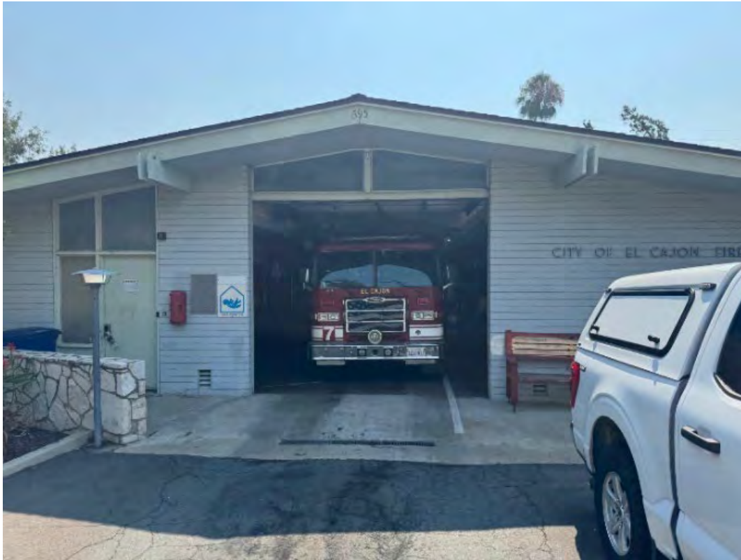
Photo 4: Fire Station No. 7 with One Bay
